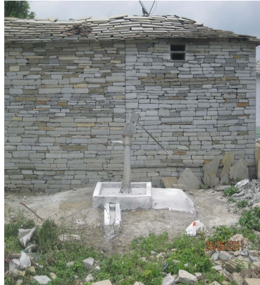
HAND PUMP ERECTED
