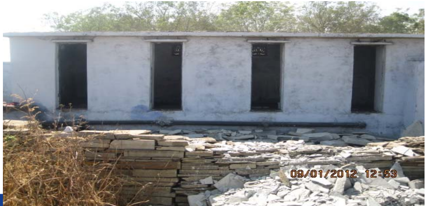
CONSTRUCTION OF TOILET FOR PUBLIC
